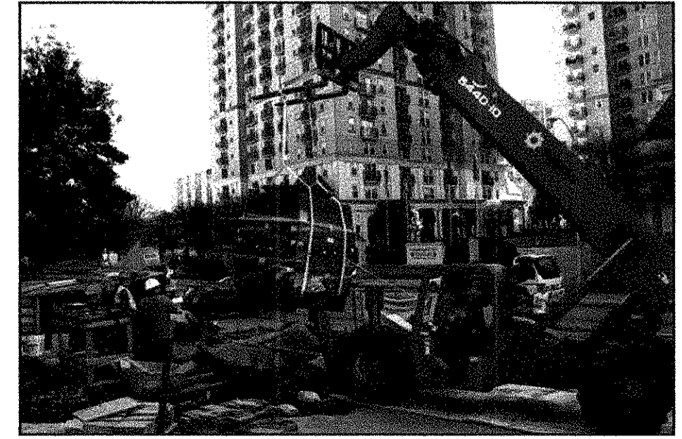
LIFTING FORK CRANE WITH DOUBLE STRAP SLING
